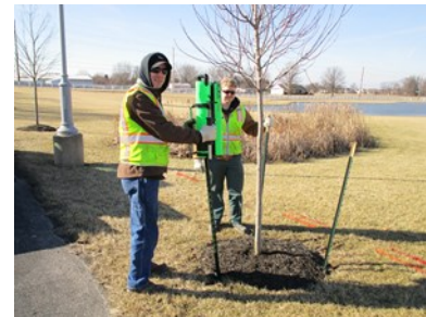
Staking trees at the service dept. driveway.
