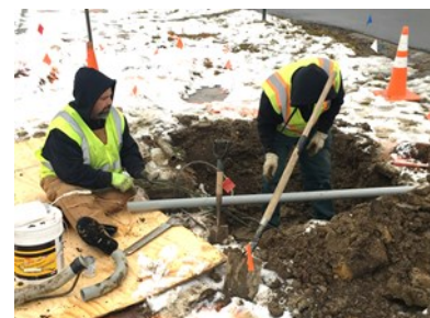
Service department crew members perform extensive underground streetlight repairs.
