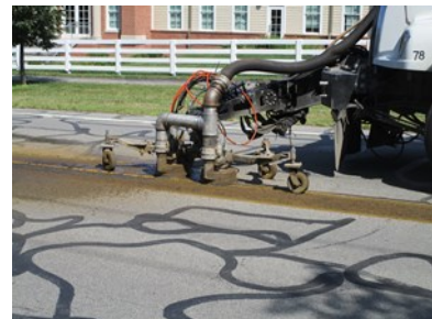
Removal of striping for application of microsurfacing.
