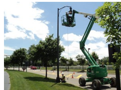
Streetlight painting is a routine task which is performed each year.
