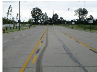
Typical roadway section designated for microsurfacing treatment.
