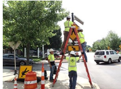
New crosswalk signals being installed and tested on Market Street.
