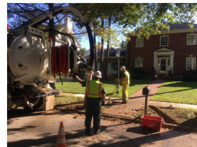
Crews install yard drains on Olmstead Rd. to alleviate ponding water on the sidewalk.
