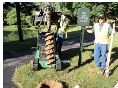
Installation of No ADA Access signs.
