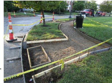
New ADA ramp at Grate Park and Gilg Street
