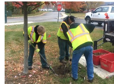
Service crews uncover a buried sanitary sewer manhole.
