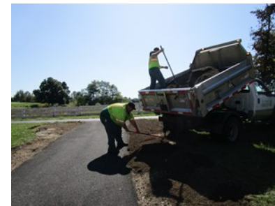
Top-soiling leisure trail on Brandon Road across from Redford Court.
