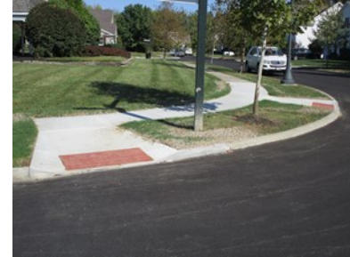
Replacement ADA Ramps and Sidewalks.
