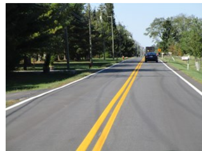
Microsurfacing was completed on Central College Road east of SR 605.
