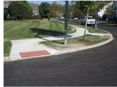
Replacement ADA Ramps and Sidewalks.
