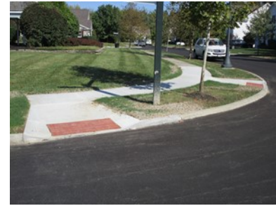
Replacement ADA Ramps and Sidewalks.
