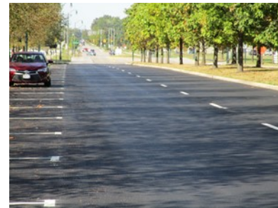
Repaved Central College Road looking West.
