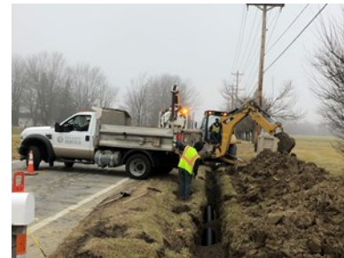
Crews install new catch basins and drainage tile on Walnut Street.
