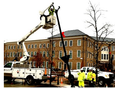
Service crews replace a streetlight damaged at Main and Market Street.
