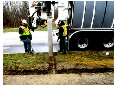
Workers use the hydro excavator to install new drain tile.
