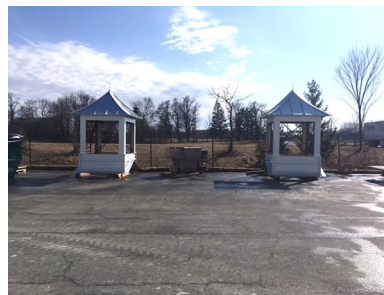
Building cupolas are built and waiting placement on the roof.
