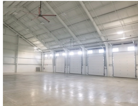
Painting contractors have completed the walls and ceiling painting.
