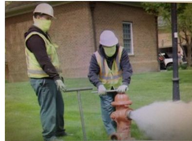
Maintenance crew Carl McNeal and Curtis Reed flushing city fire hydrants.
