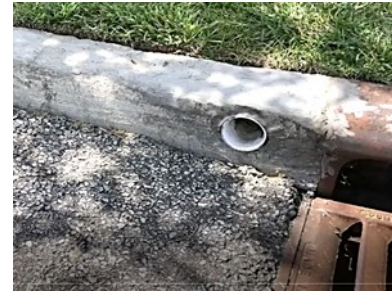
Curb repaired at Straights Farm.
