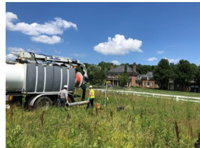
Sanitary Sewer cleaning in the New Albany Farms
