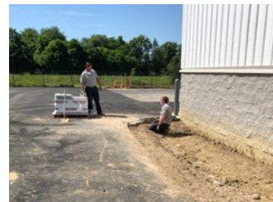
Crews work to install a landscape retaining wall outside the addition.
