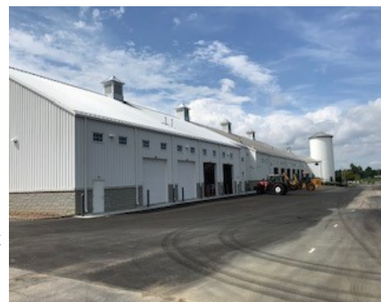
Lot paving was completed to the Service Garage Addition.
