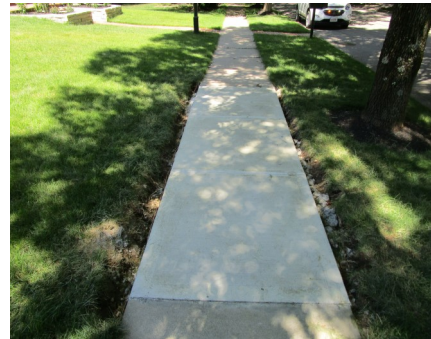
Sidewalk form boards have been removed and topsoil is to be placed.
