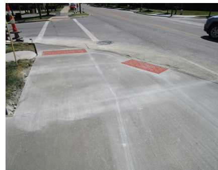
New ADA ramp at Village Hall Rd. and Johnston Rd.
