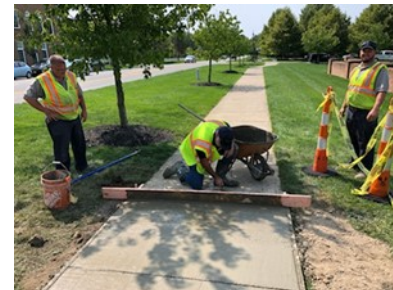
Service crews replace two bad sidewalk panels on Johnstown Road.
