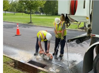
Crews perform catch basin repair on New Albany Road East.
