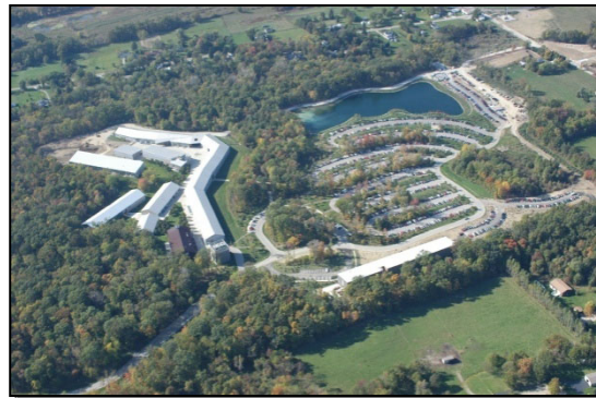
Figure 6 – Aerial View of Business Campus
