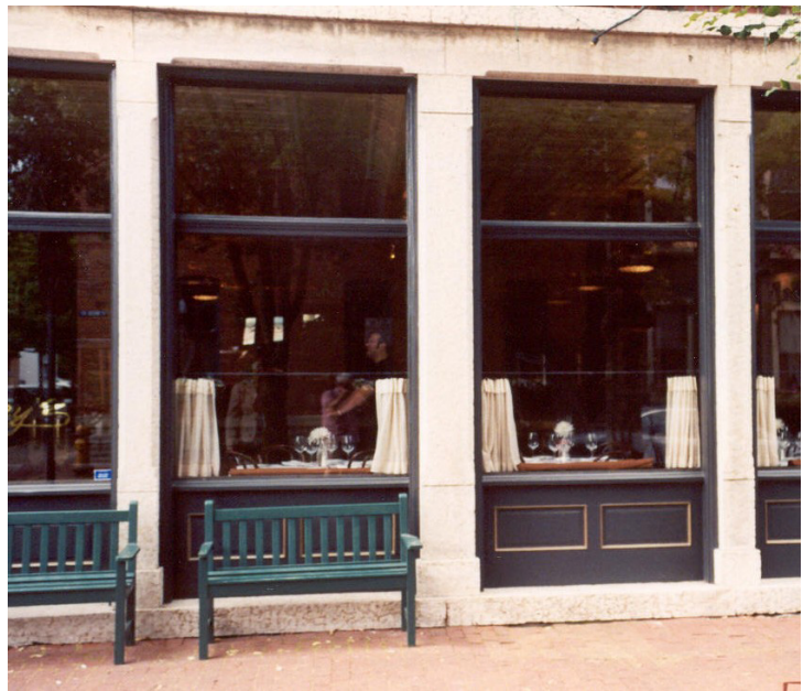
Storefront display windows typically had large panes of glass rather than smaller divided light glazing found in residential designs.
