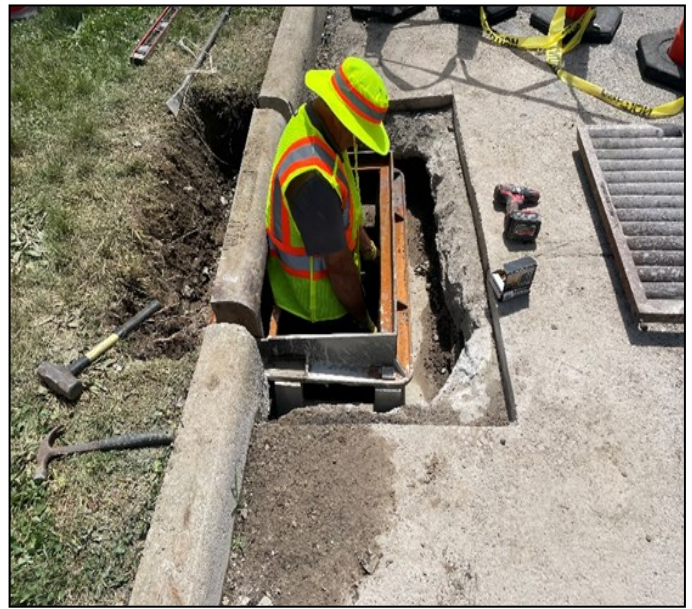
Dave Thatcher, Kerry Gastaldo, Keith Unterbrink, Christian Duane, and Nick Sgandurra all working on repairing the catch basin on Griswold Dr.
