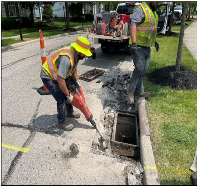
Dave Thatcher, Kerry Gastaldo, Keith Unterbrink, Christian Duane, and Nick Sgandurra all working on repairing the catch basin on Griswold Dr.
