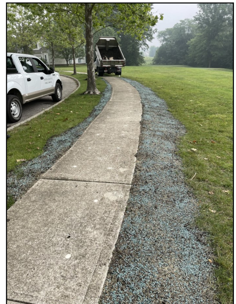
Right of way crew laying topsoil and seed at Decker and Jersey Drive
