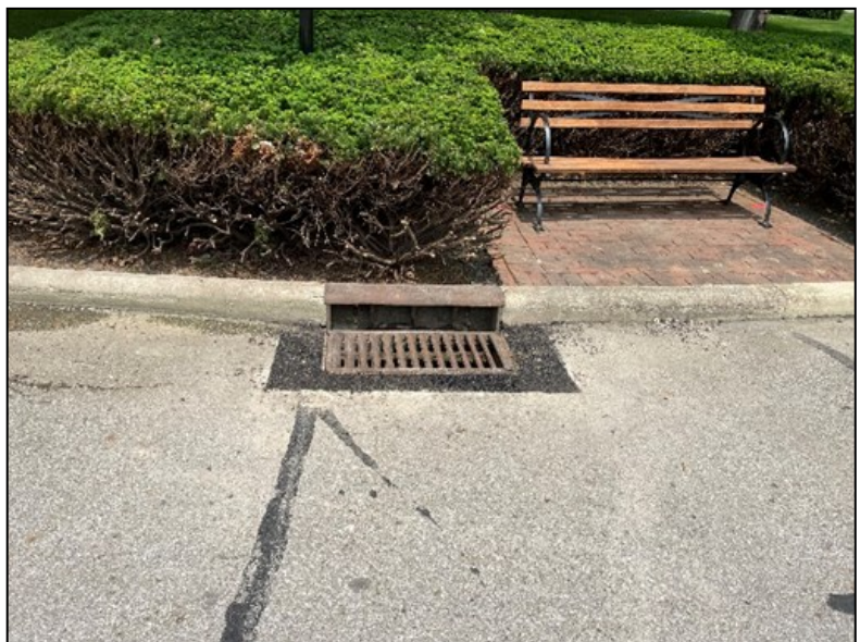
One of the completed basin structures
