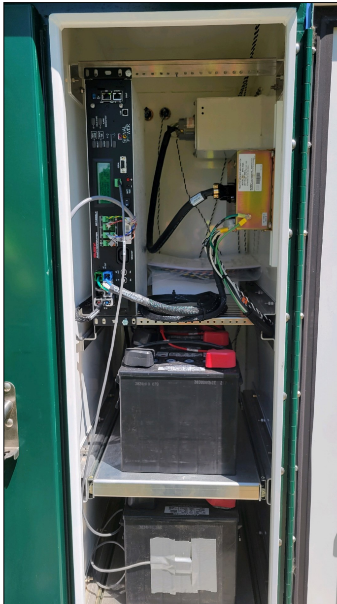
UPS cabinet with the clary back-up controller and batteries
