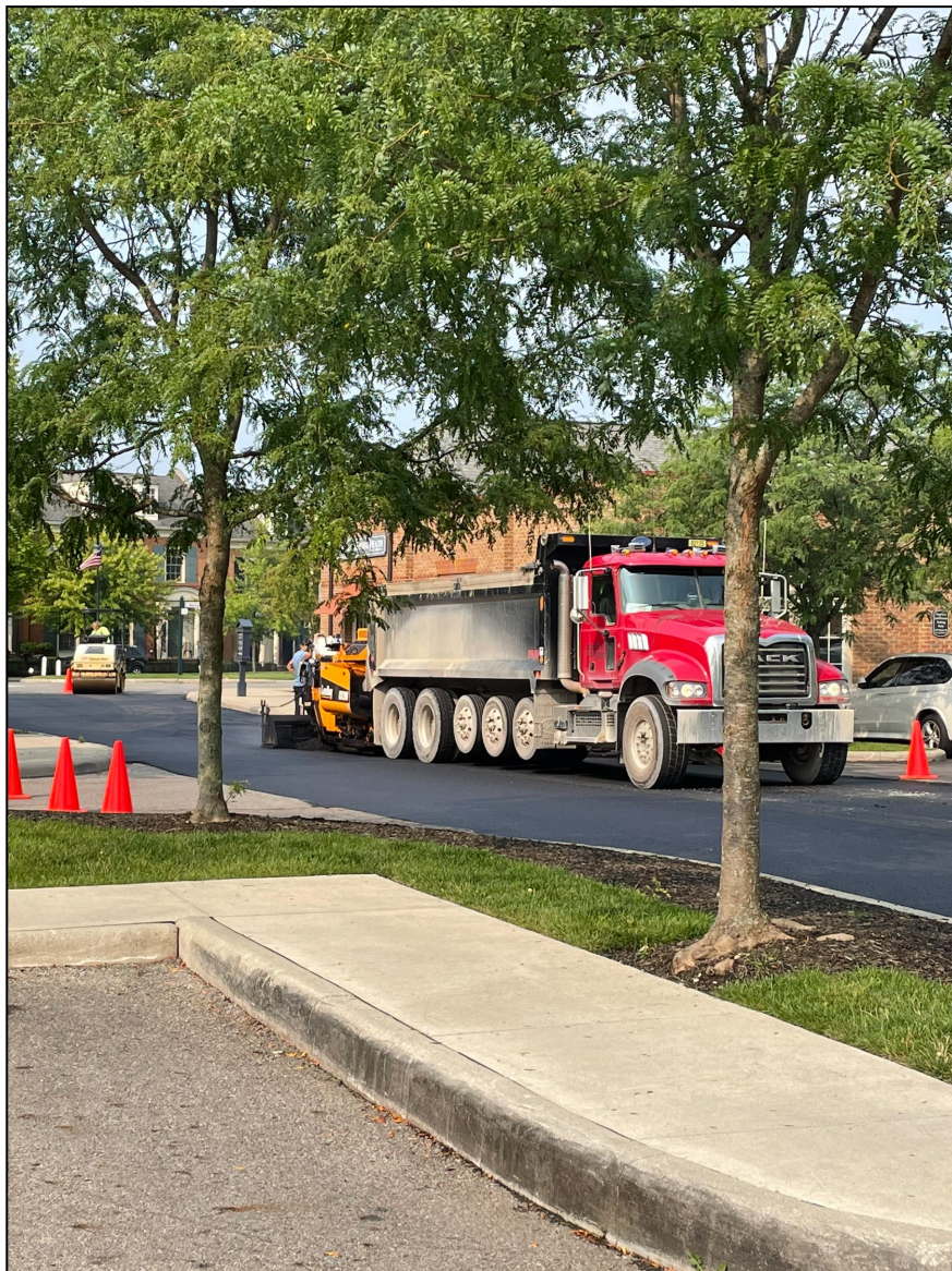
Seal coating being applied at the Heit Center
