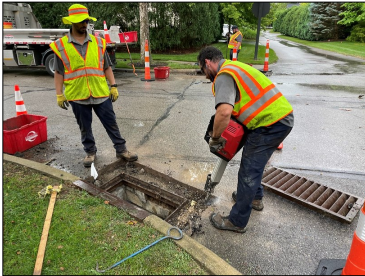
Nick Sgandurra and Kerry Gastaldo removing existing brick around the basin.
