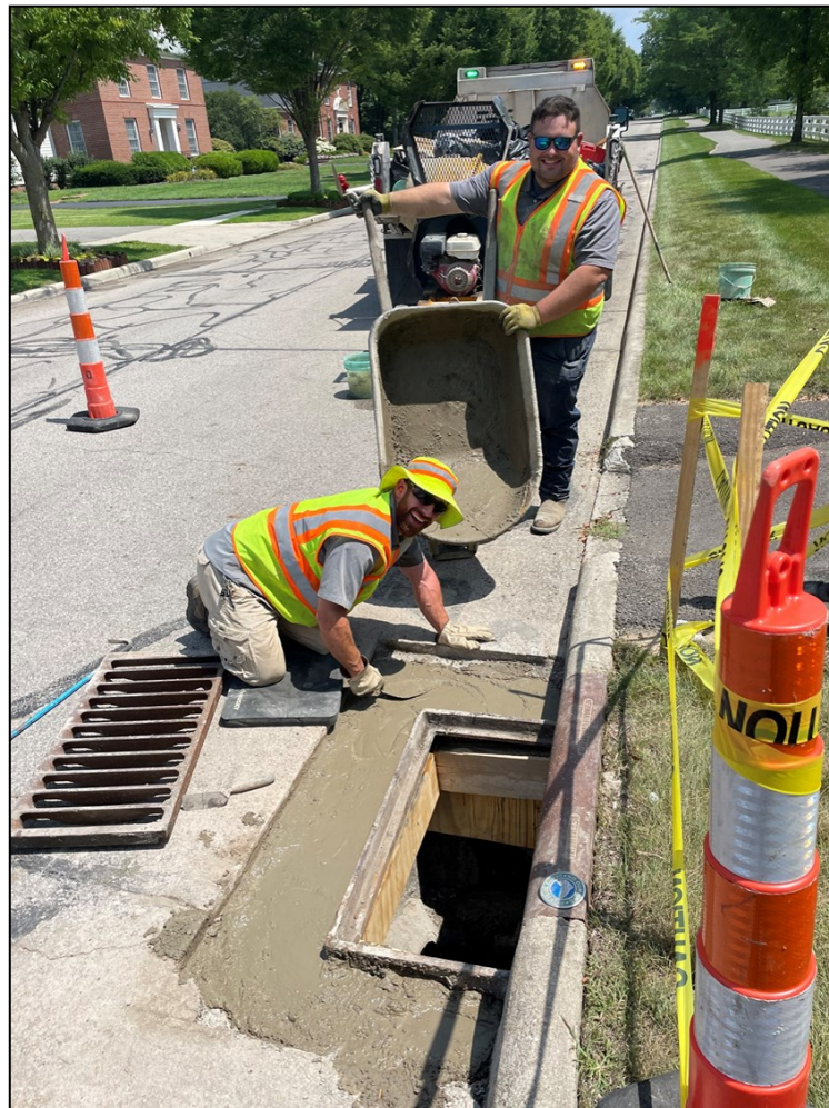
Maintenance workers Christian Duane and Nick Sgandurra put the finishing touches on a reconstructed curb inlet
