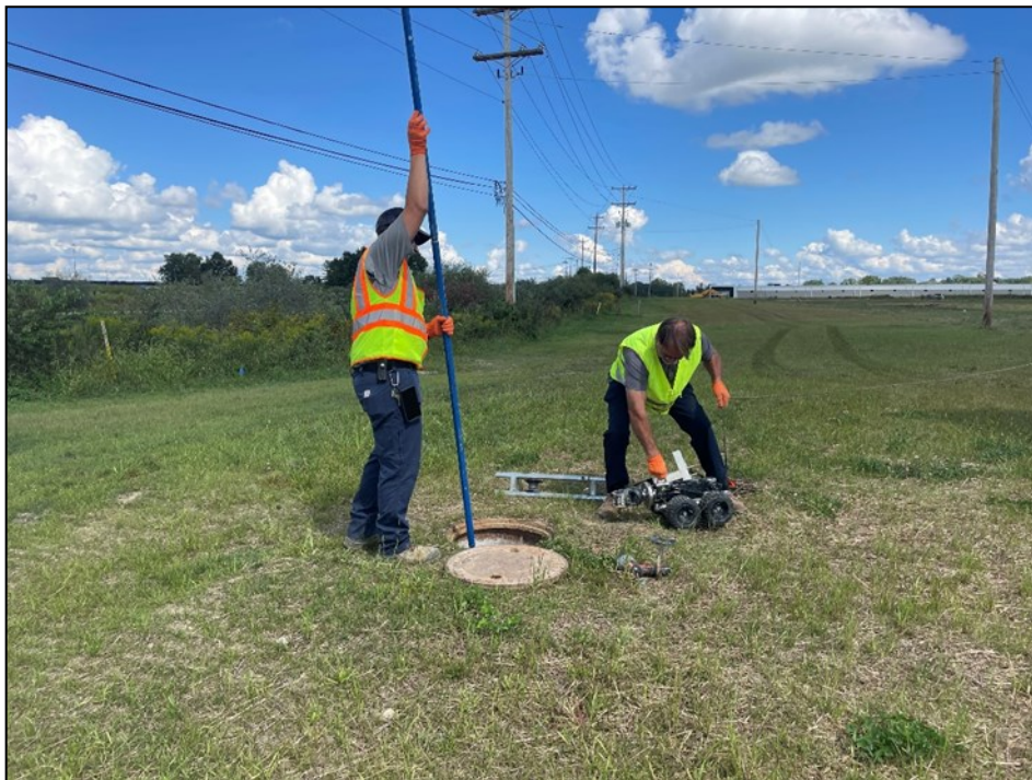
David Thatcher and Kerry Gastaldo setting up sanitary line inspection.
