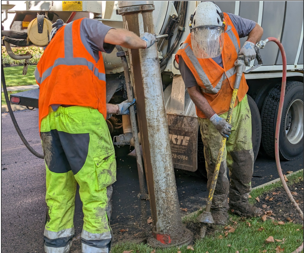
Sam Darnall and Chase Loughman use a combination of the vac truck and airspade to safely excavate around the large roots of London plane trees on Holkham.
