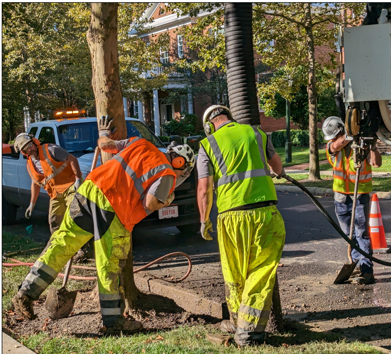
Curtis Reed, Sam Darnall, Chase Loughman, and Nick Sgandurra use the vac truck and airspade to excavate and prune roots on Holkham.
