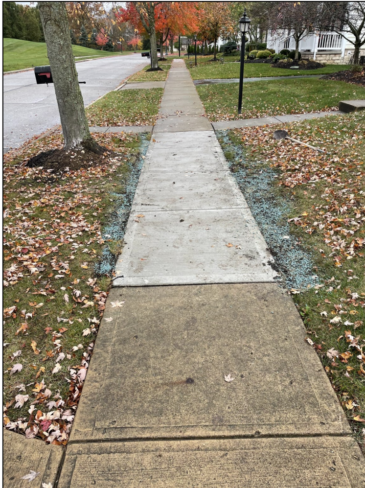
Fully restored sidewalk leveling
