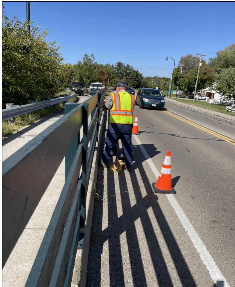
Crew members Carl McNeal, Mike Cligrow and Rick Goldhardt seen installing the fourth rail along the bridge.
