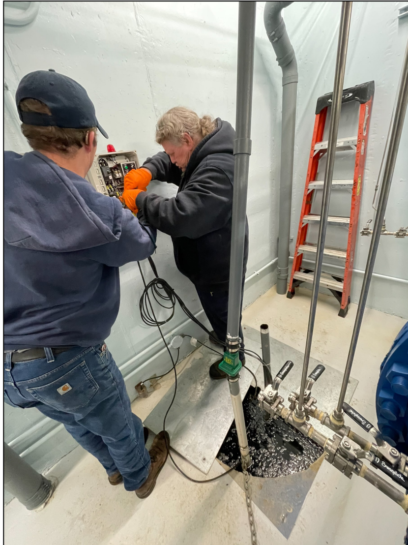
Jerry Smith and Tyler Myers wiring up replacement grinder pump at booster station on Morse Rd.
