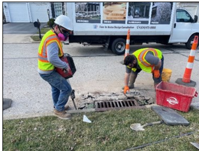
Tommy Diamond and Christian Duane jackhammering the frame to rebuild the cement surrounding storm drain curb inlet
