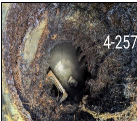
Left: Inside a sanitary sewer manhole structure 12" below the existing grade Right: Sanitary sewer structure from street view
