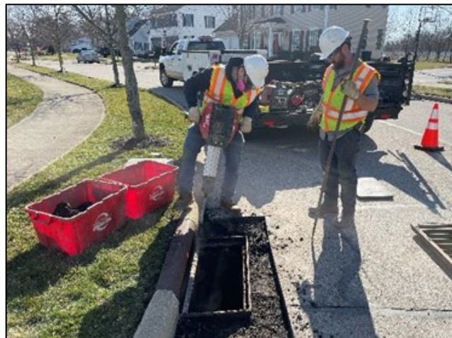
Tommy Diamond and Nick Sgandurra fixing the cement around storm drain curb inlet
