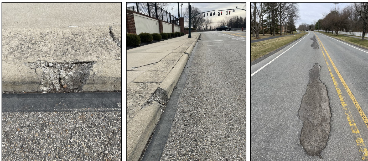
Left and center: Examples of curbs in need of curb replacement
