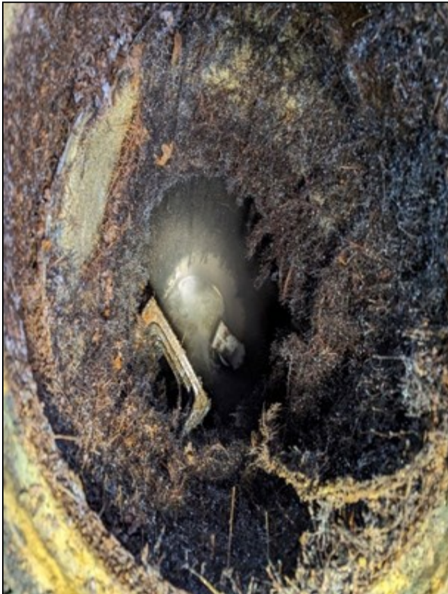
Left: Before picture of sanitary sewer with roots Right: After picture of the sanitary sewer after root removal and liner application took place
