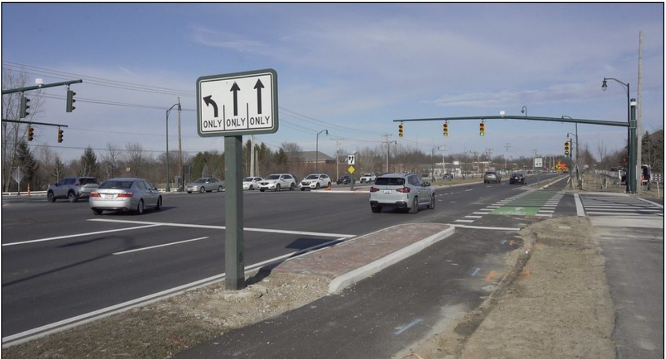
Signalized intersection at SR-161 and US 62
