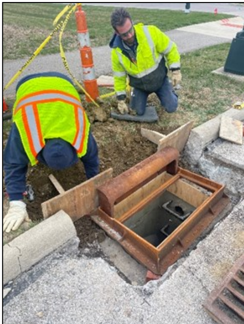
Maintenance worker Nick Sgandurra and seasonal maintenance worker John Mikulec gather measurements while installing a new curb inlet frame
