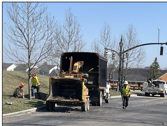
Tree removal on SR-605
