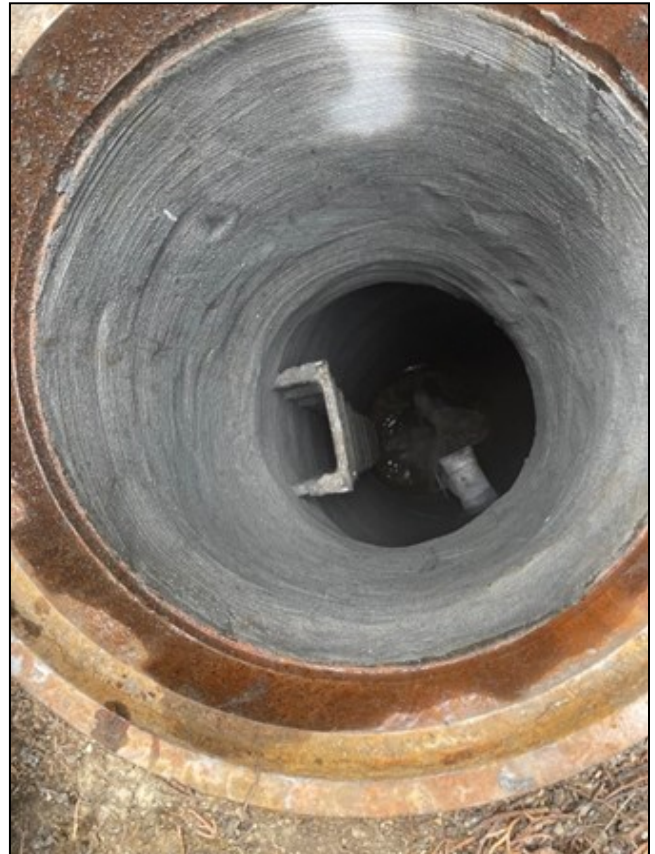
Left: Before picture of sanitary sewer with roots Right: After picture of the sanitary sewer after root removal and liner application took place
