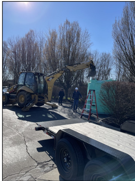
Village Hall water tank delivery
