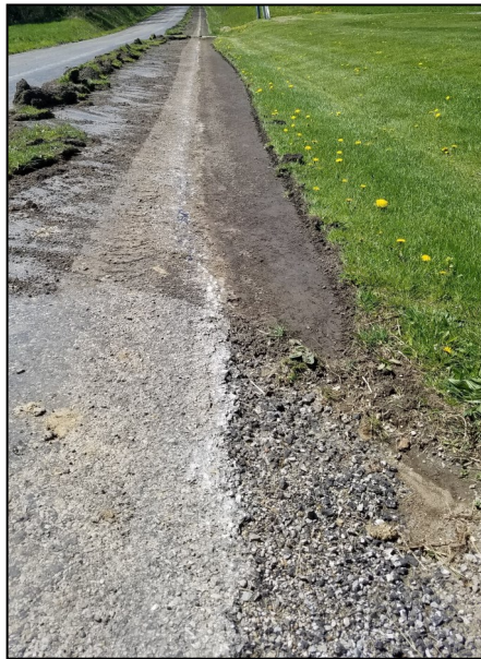
Left: Berm in need of restoration
