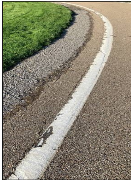
Left: Berm in need of restoration
