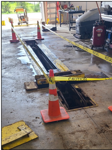
In-ground lift after being striped for repair
