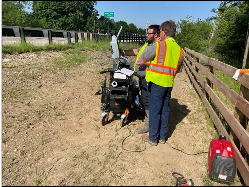
Inspecting the sanitary sewer pipe that serves Taylor Farm Park
