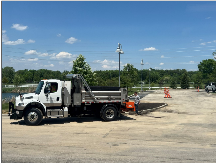
Tyler Myers and Tommy Diamond backfilling the new curb
