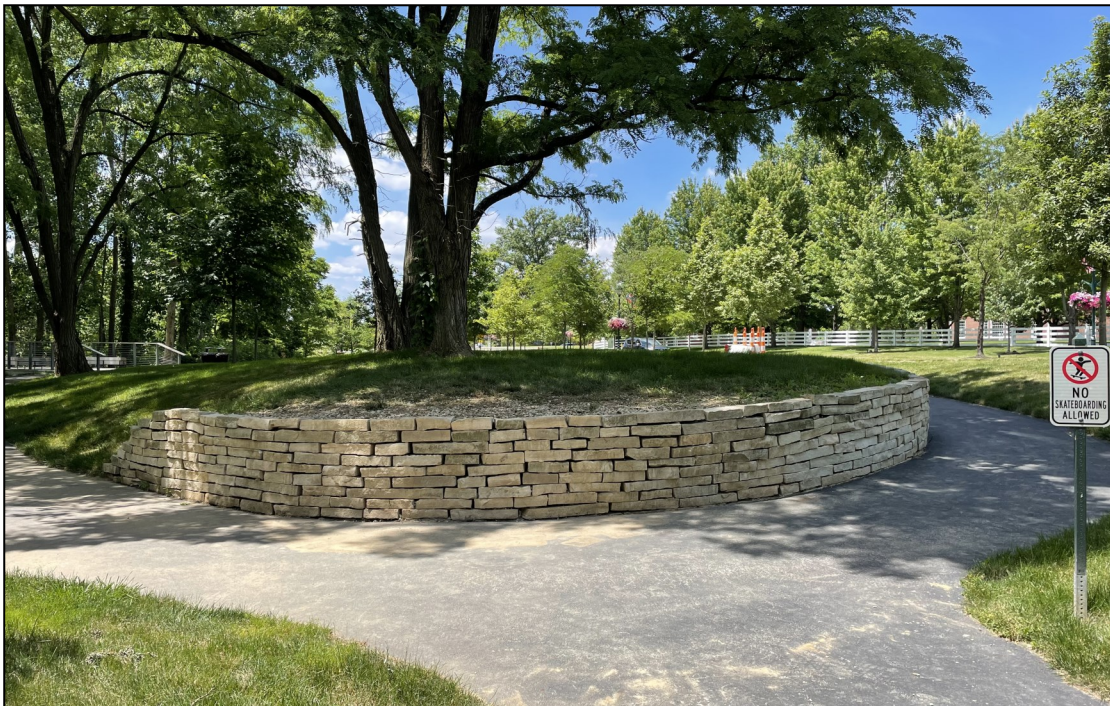
Restoration of stone wall completed
