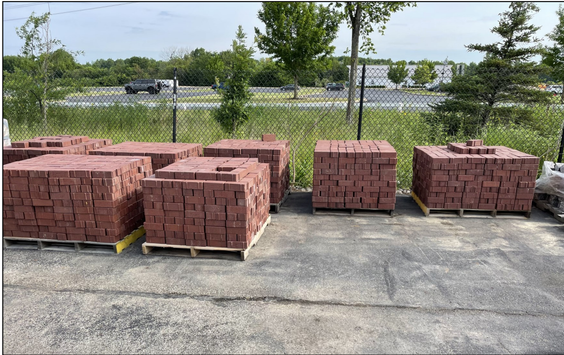
Brick paver inventory was taken
