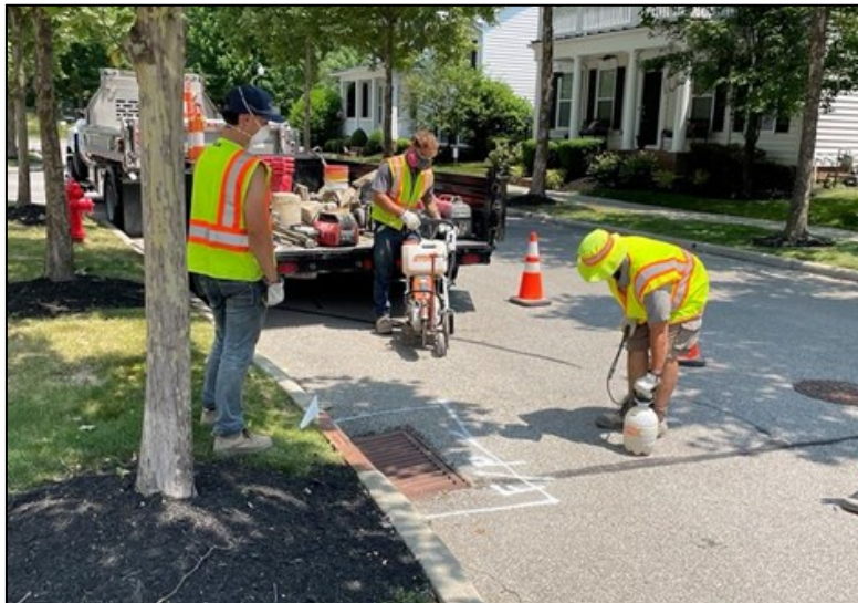
Kerry Gastaldo, Tommy Diamond and Maxwell Deckop working on a Blackstone Edge Dr. curb inlet
