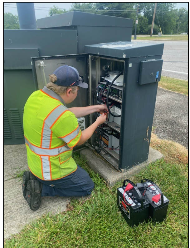
Ian Hurst replacing the batteries and running a test on the intersection
