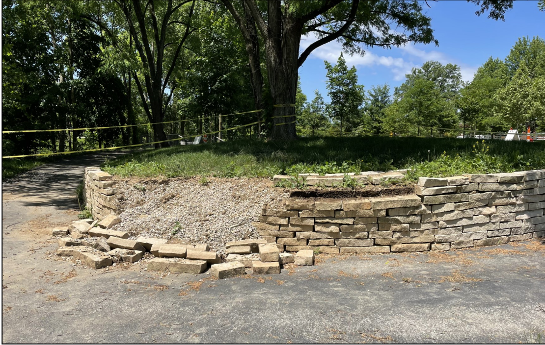
Before stone wall was restored
