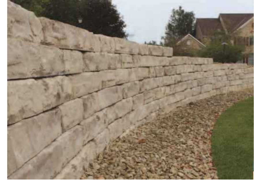
Low Wall at Bioretention Basin. Dry-laid, stone look concrete masonry wall, Oberfields Kodah or Similar.
