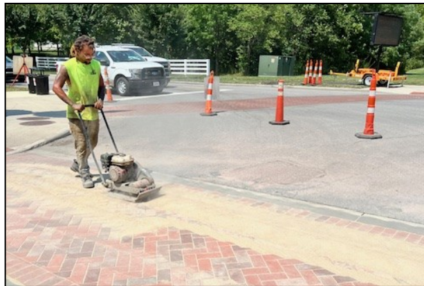
Adding sand to fill in gaps and smoothing the crosswalk
