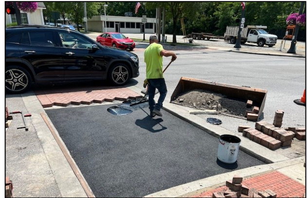
Bituminous layer being placed
