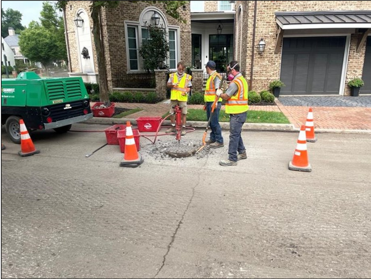
Maintenance workers Nick Sgandurra, Tommy Diamond and David Thatcher resetting a sanitary manhole frame on Hays Town
