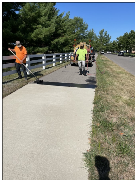
Left: Before resealing leisure trail Right: After resealing pathway
