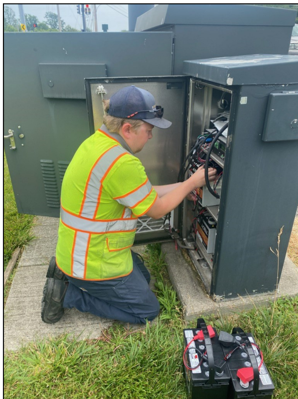
Ian Hurst replacing the batteries and running a test on the intersection
