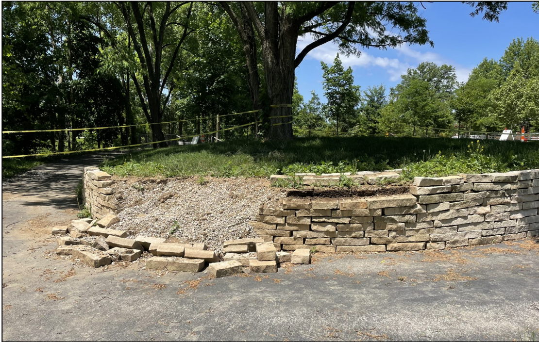
Before stone wall was restored
