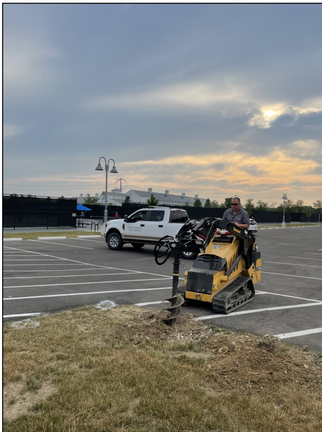
Left: Boring holes for new fencing Right: Fencing finished at pickleball facility
