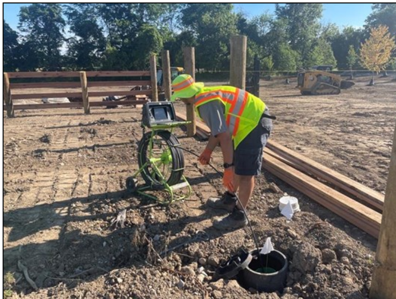
Kerry Gastaldo performing a CCTV inspection of the sanitary service lines
