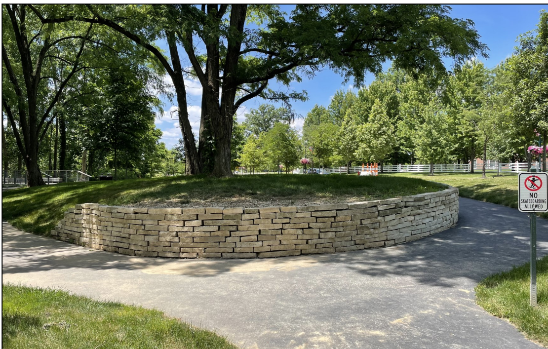
Restoration of stone wall completed
