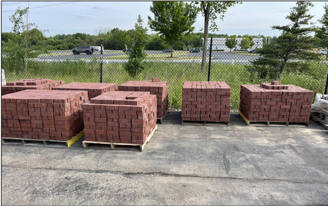
Brick paver inventory was taken
