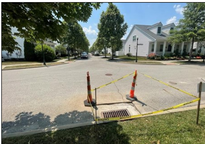
Curb inlet completed
