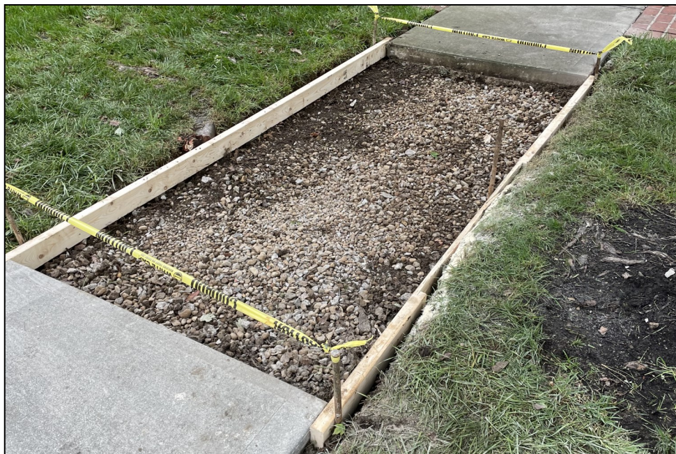
Sidewalk panel removed and prepped for new cement to be poured
