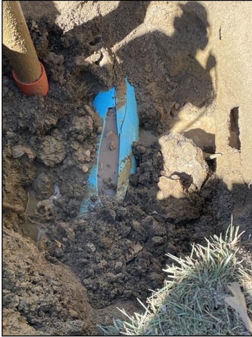
Left: Complete General excavating down to the 15" pipe Right: Uncovering the broken pipe
