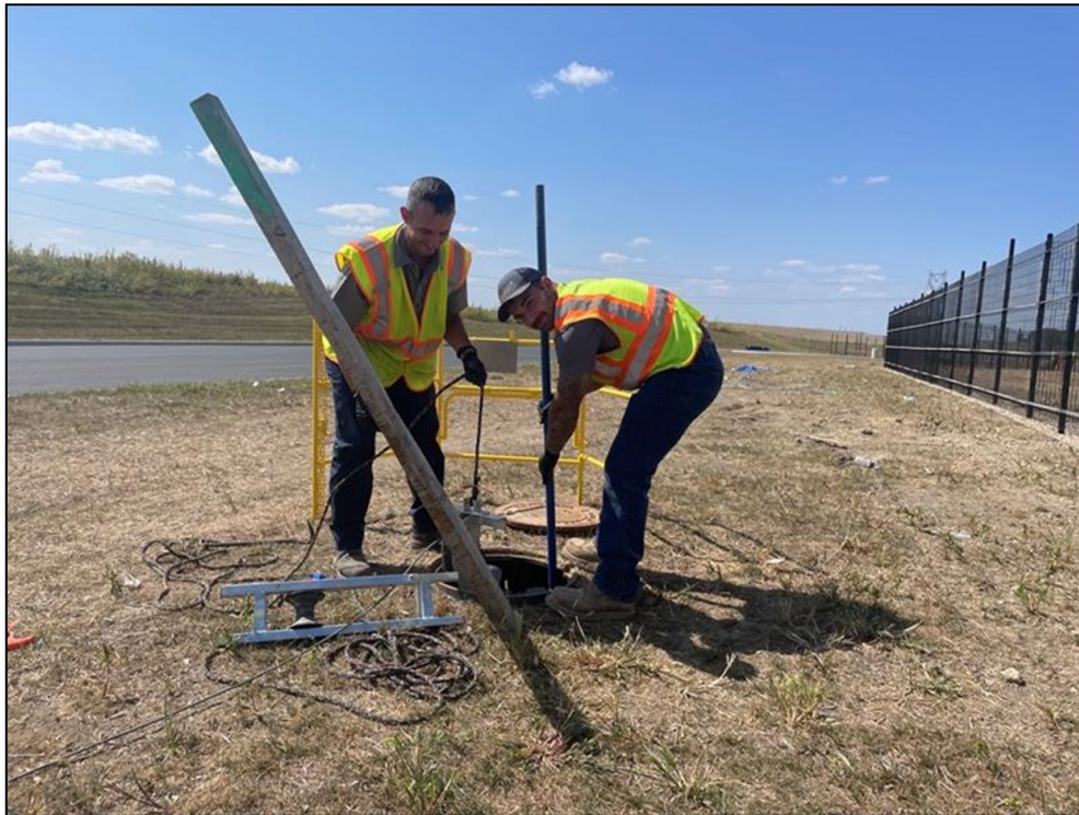
Tommy Diamond and Kerry Gastaldo conducted a pre-acceptance CCTV survey of the BTS sanitary sewer main lines
