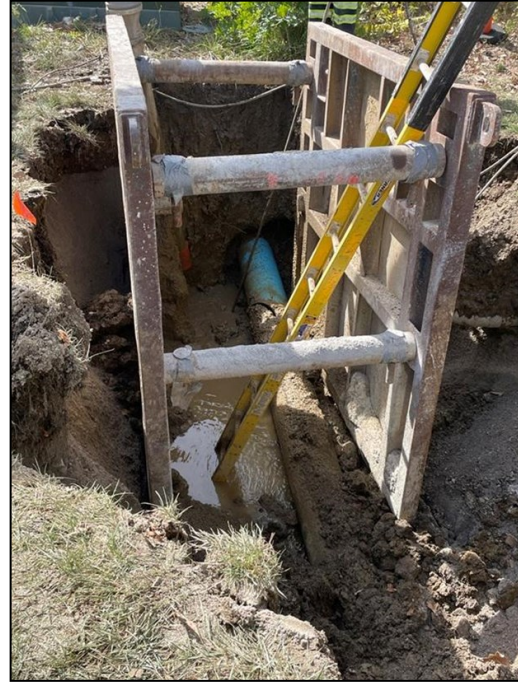
Left: Complete General excavating down to the 15" pipe Right: Uncovering the broken pipe
