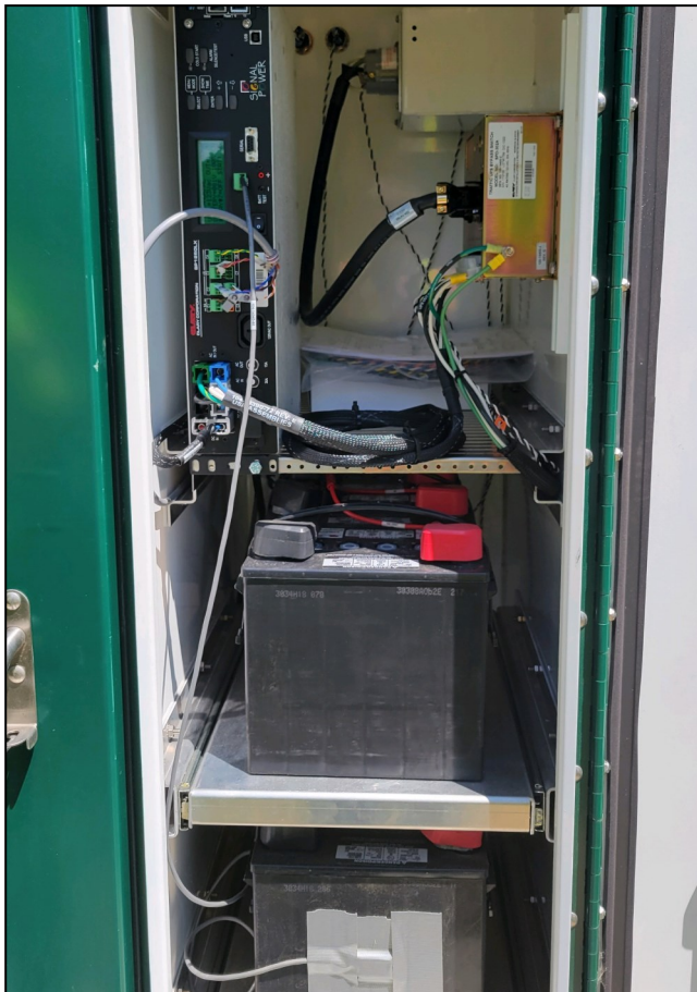
Left: Cabinet with batteries engaged Right: Ian Hurst is checking voltage on the UPS batteries, making sure they are within tolerance
