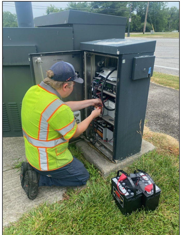
Left: Cabinet with batteries engaged Right: Ian Hurst is checking voltage on the UPS batteries, making sure they are within tolerance
