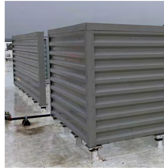
Rooftop Screening material: corrugated metal manufacturer: tbd style: horizontal color: match FC-3
