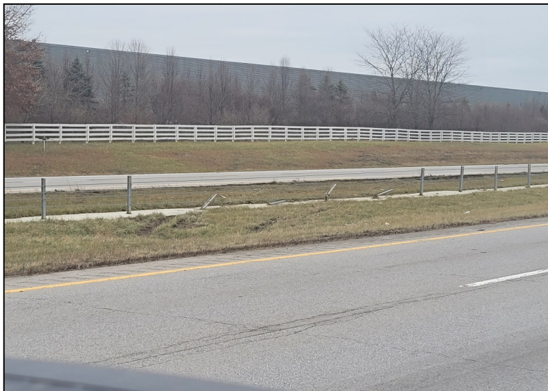
Cable guardrail along SR-161 prior to replacement
