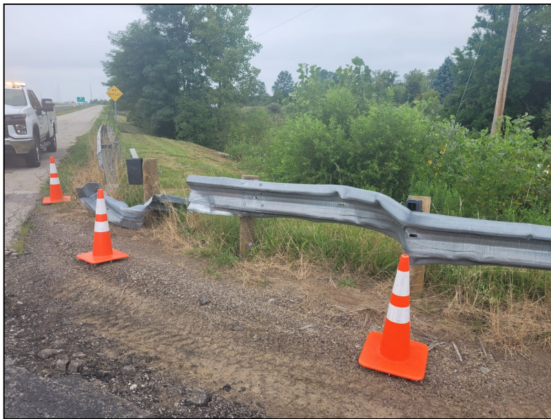
Galvanized channel guardrail prior to replacement along E Dublin-Granville Rd.
