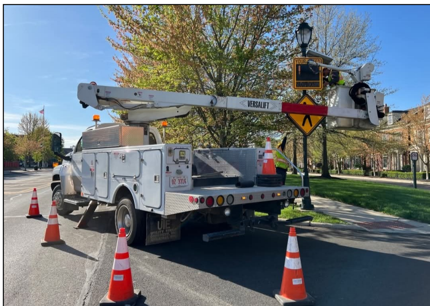
Shaun Bush in bucket truck securing speed feedback sign along Market St.
