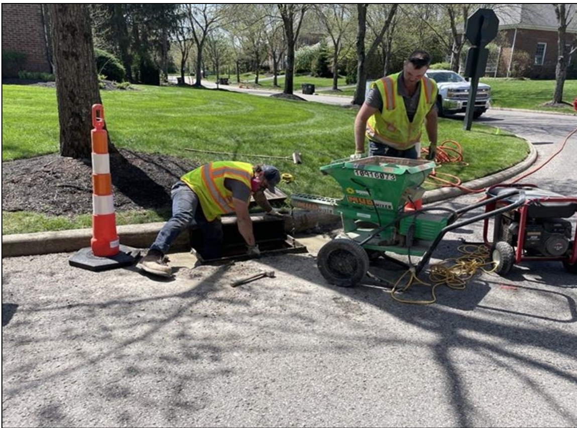
Daitan Rood and Tommy Diamond reconstructing a basin structure on Farber Ct.
