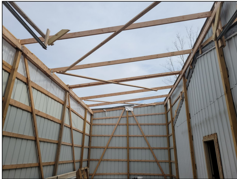
Structure without the roof due to high winds
