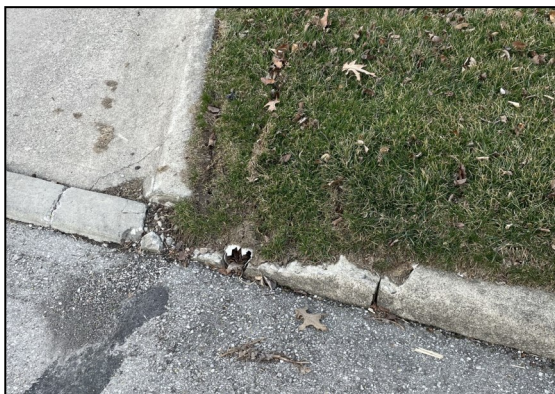
Left and Right: Crumbling curbs around the city
