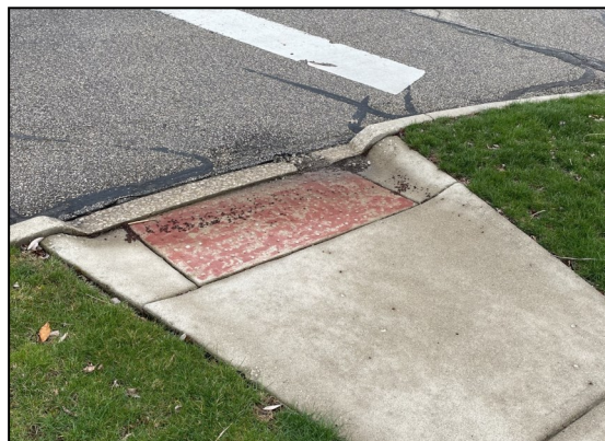
Left and Right: Non-compliant ADA ramps
