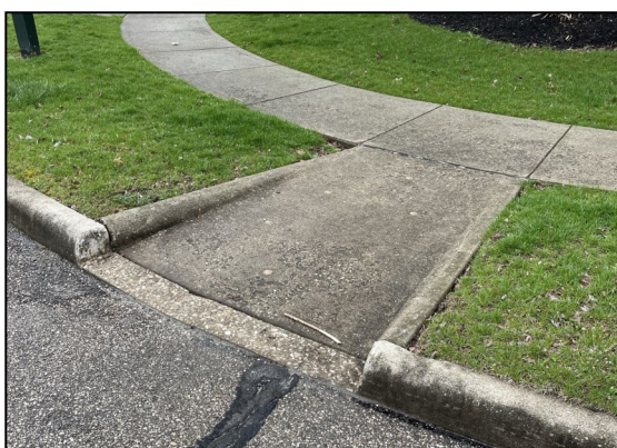
Left and Right: Non-compliant ADA ramps
