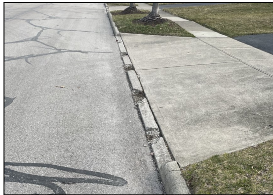
Left and Right: Crumbling curbs around the city
