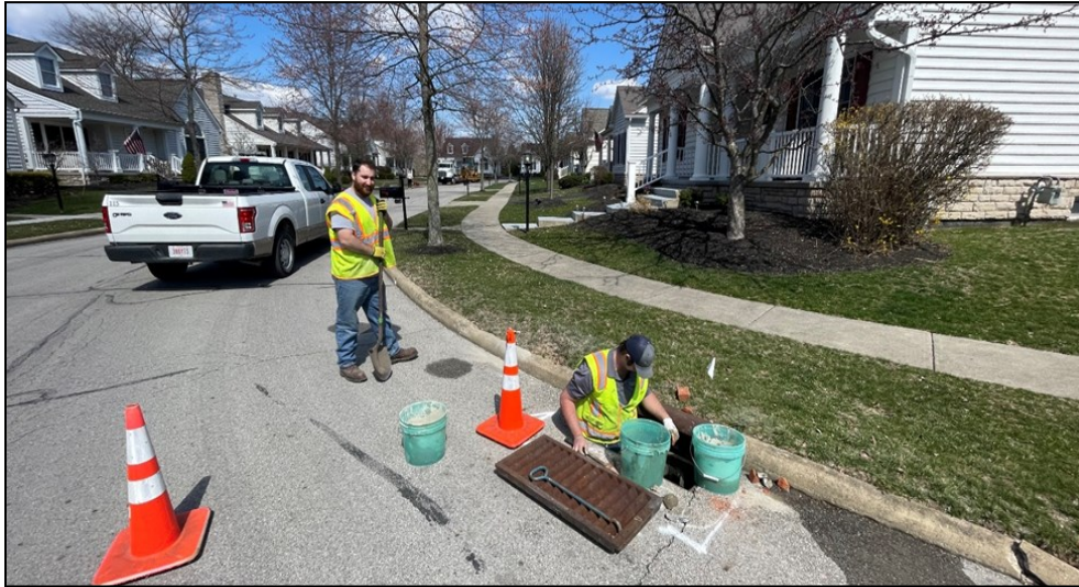
Daitan Rood and Blake Crow make repairs to a curb inlet on Keesee Circle
