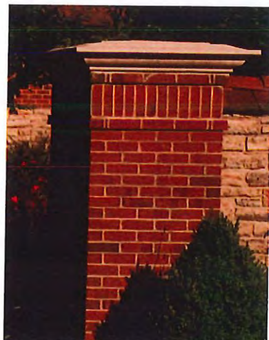
PIERS AND SITE WALL
