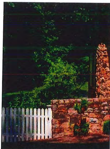
FENCE AND SITE WALL
