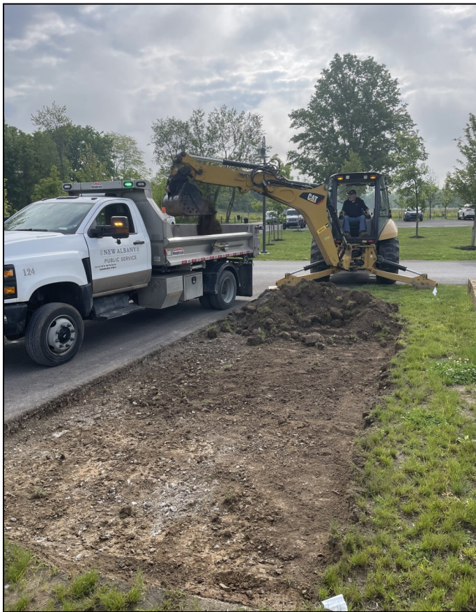
Left and right: Steve Kidwell digging up grass to place concrete for bike share at Taylor Farm Park
