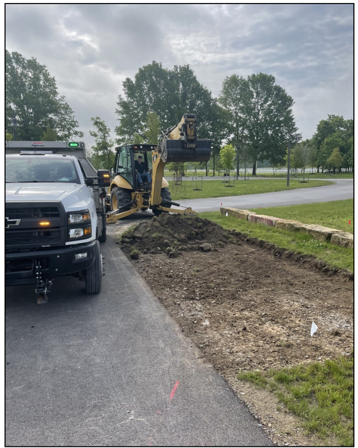
Left and right: Steve Kidwell digging up grass to place concrete for bike share at Taylor Farm Park
