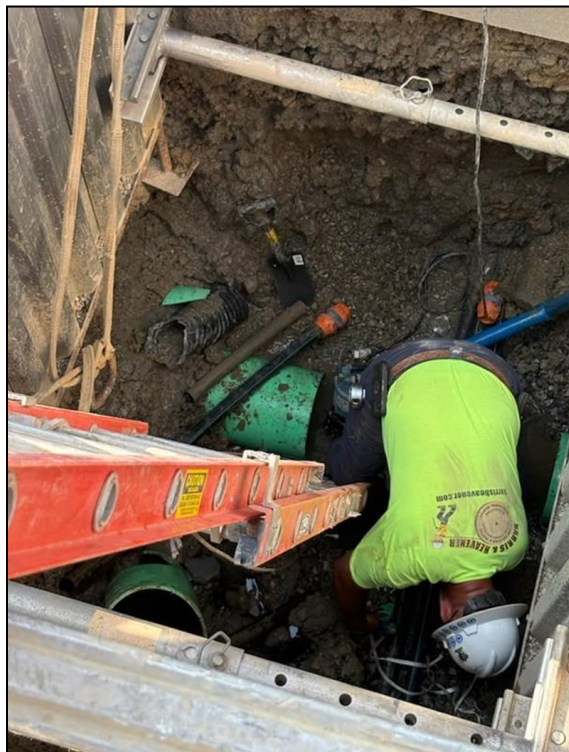
Left: 12" sanitary sewer main line damage Right: Utility duct relocation
