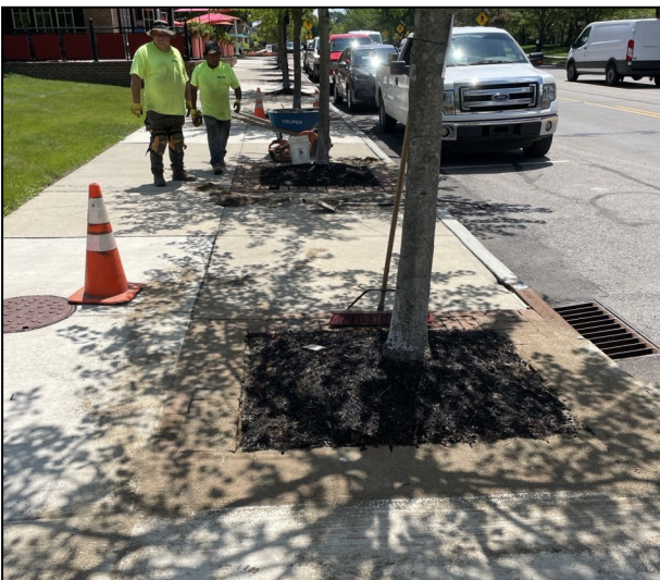
Left and Right: Brickwork being completed on tree wells throughout the village center
