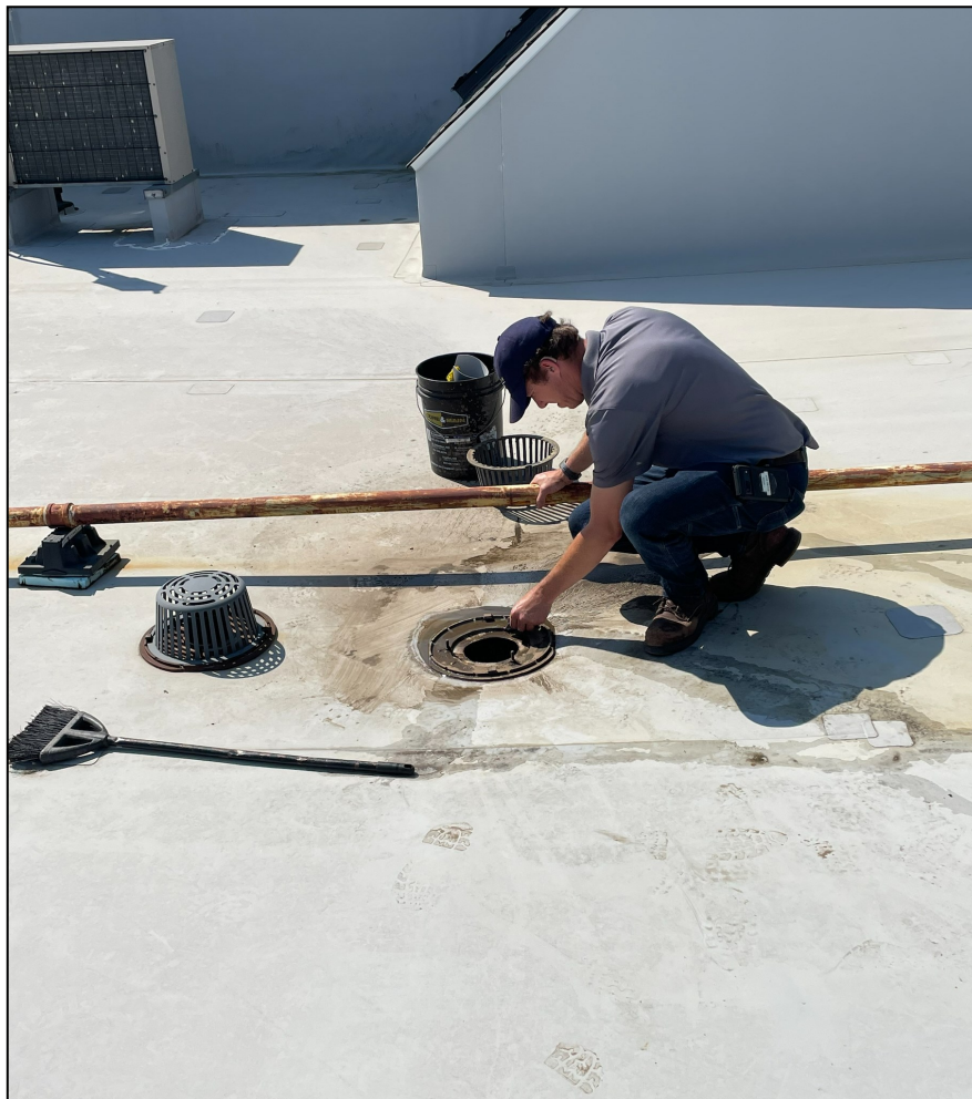
Tyler Myers clearing out the Heit Center roof drain
