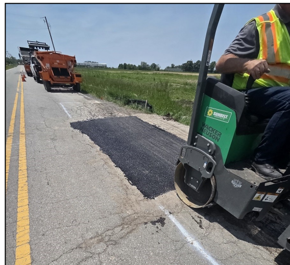
Left: After Kenny Geiger and Keith Unterbrink stamped perma-patch Right: Dennis Munsey rolling perma-patch
