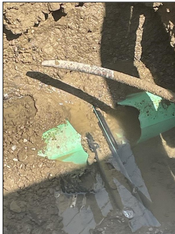
Left: 12" sanitary sewer main line damage Right: Utility duct relocation
