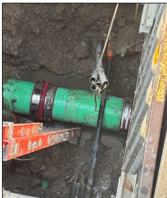
12" sanitary sewer line repaired
