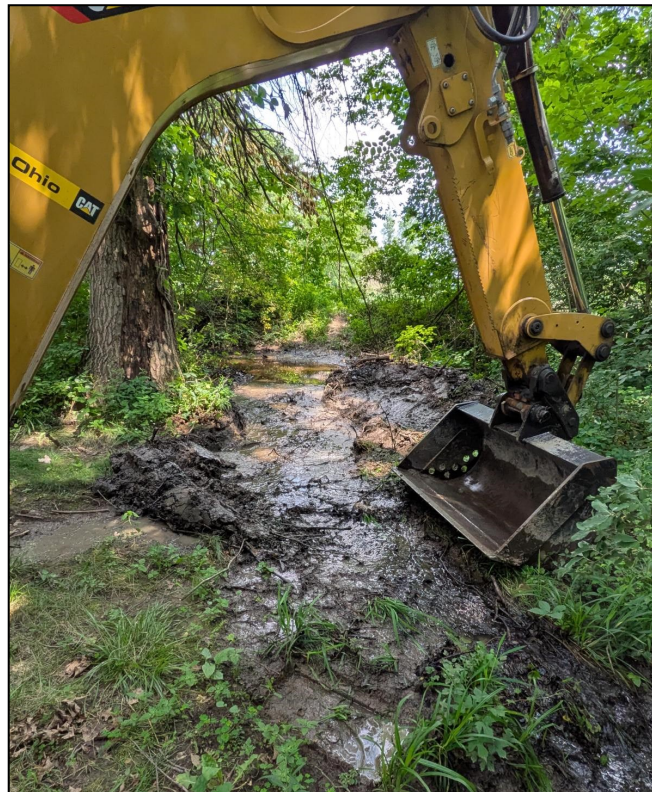
Matt Lycans and Daitan Rood removing debris from retention pond with the backhoe
