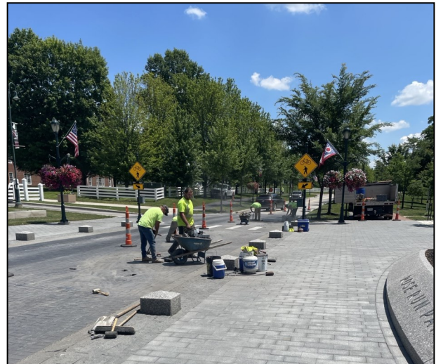
Left and Right: Brickwork being completed on Raines Crossing
