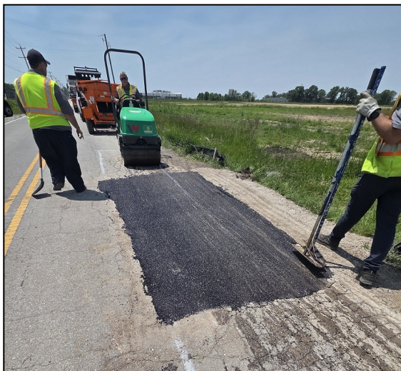
Left: After Kenny Geiger and Keith Unterbrink stamped perma-patch Right: Dennis Munsey rolling perma-patch
