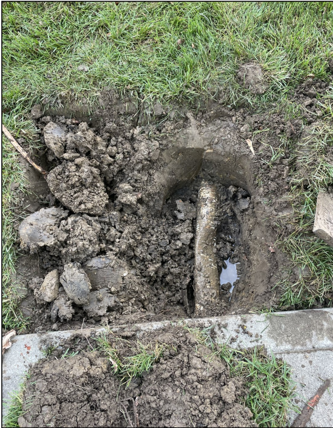
Left: Sump pump pipe before restoration
