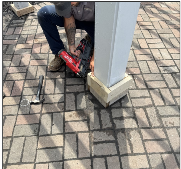
Left and right: Nate Fravel made repairs to all wood trim at the base of the pergolas
