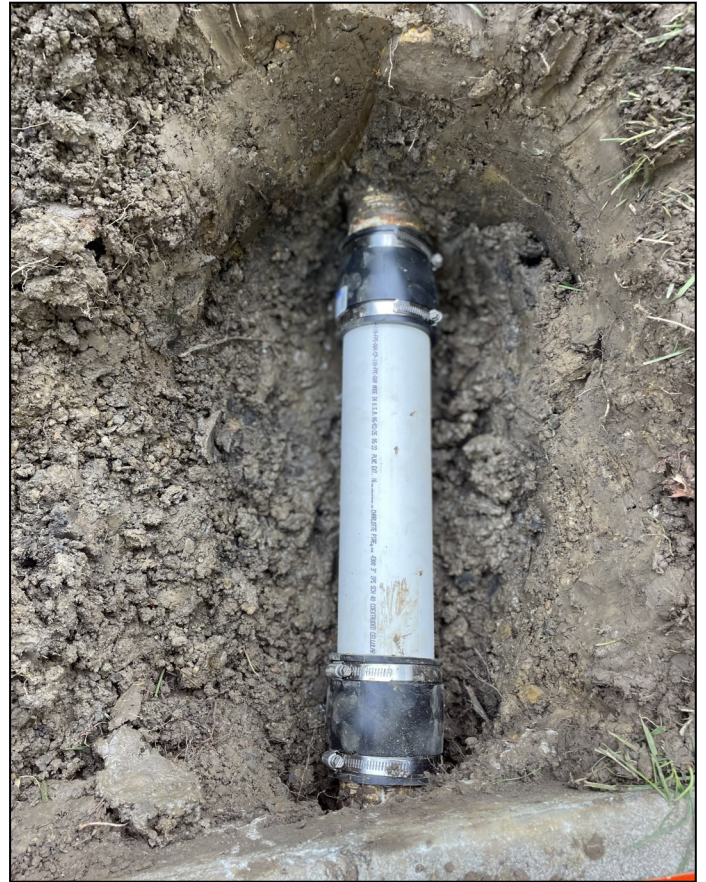
Left: Sump pump pipe before restoration
