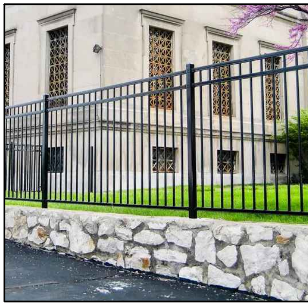
POOL FENCE: AMERISTAR MONTAGE PPP; 48" HT.
