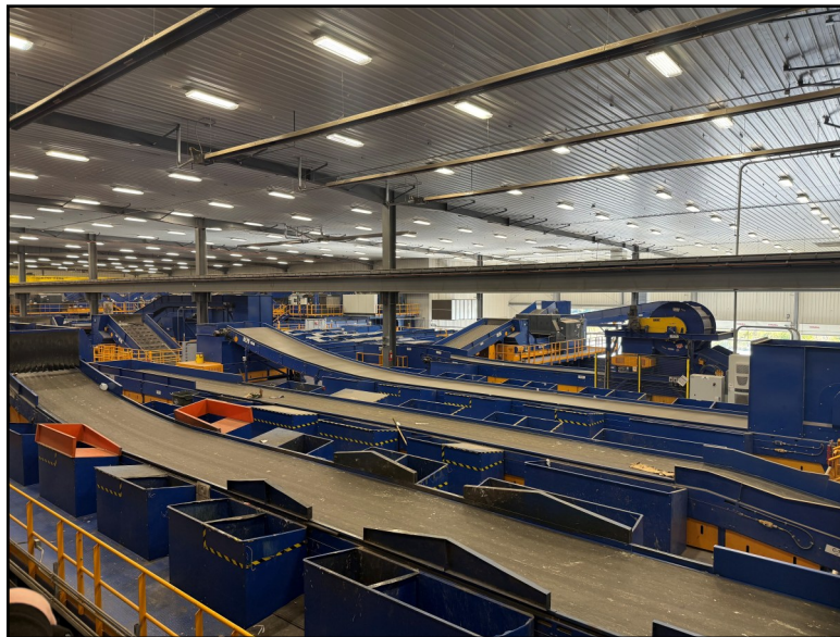
Picture from inside the facility
