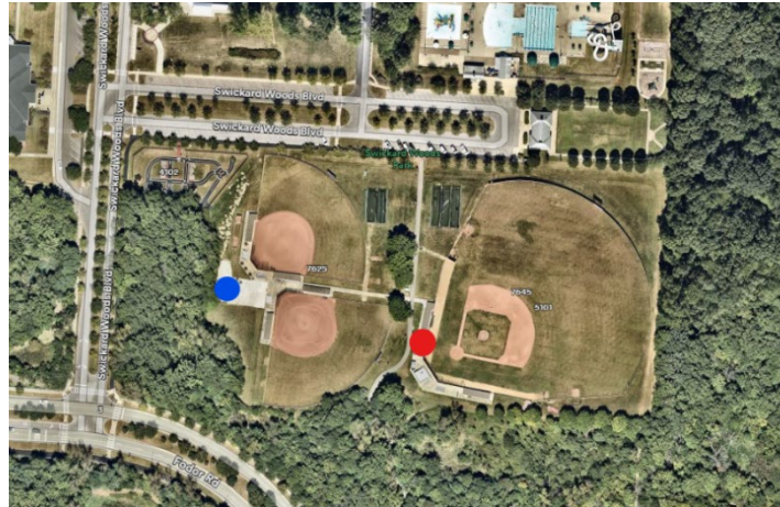
Image: existing location of storage structure (blue circle) and press box (red circle).
