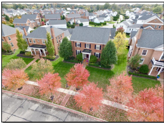
Figure 3 – Example of Residential Architecture
