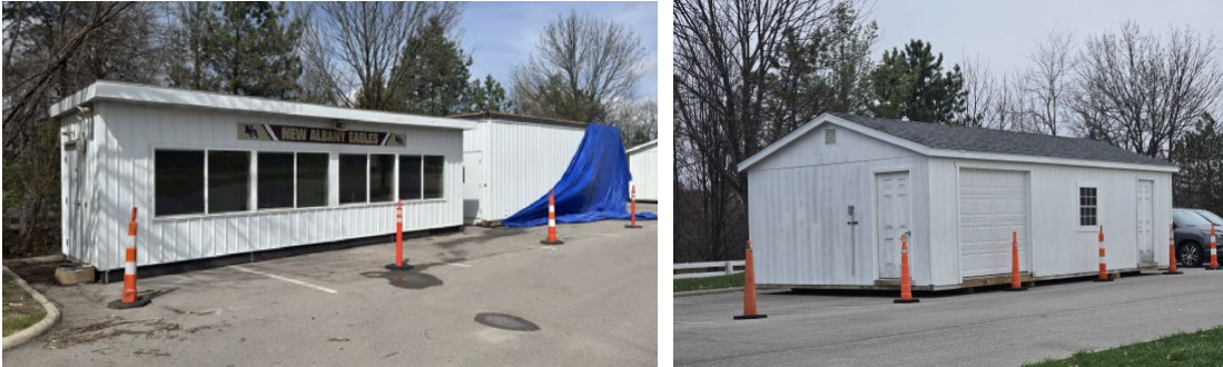
Images: press box (left), to be stacked, and storage structure (right).
