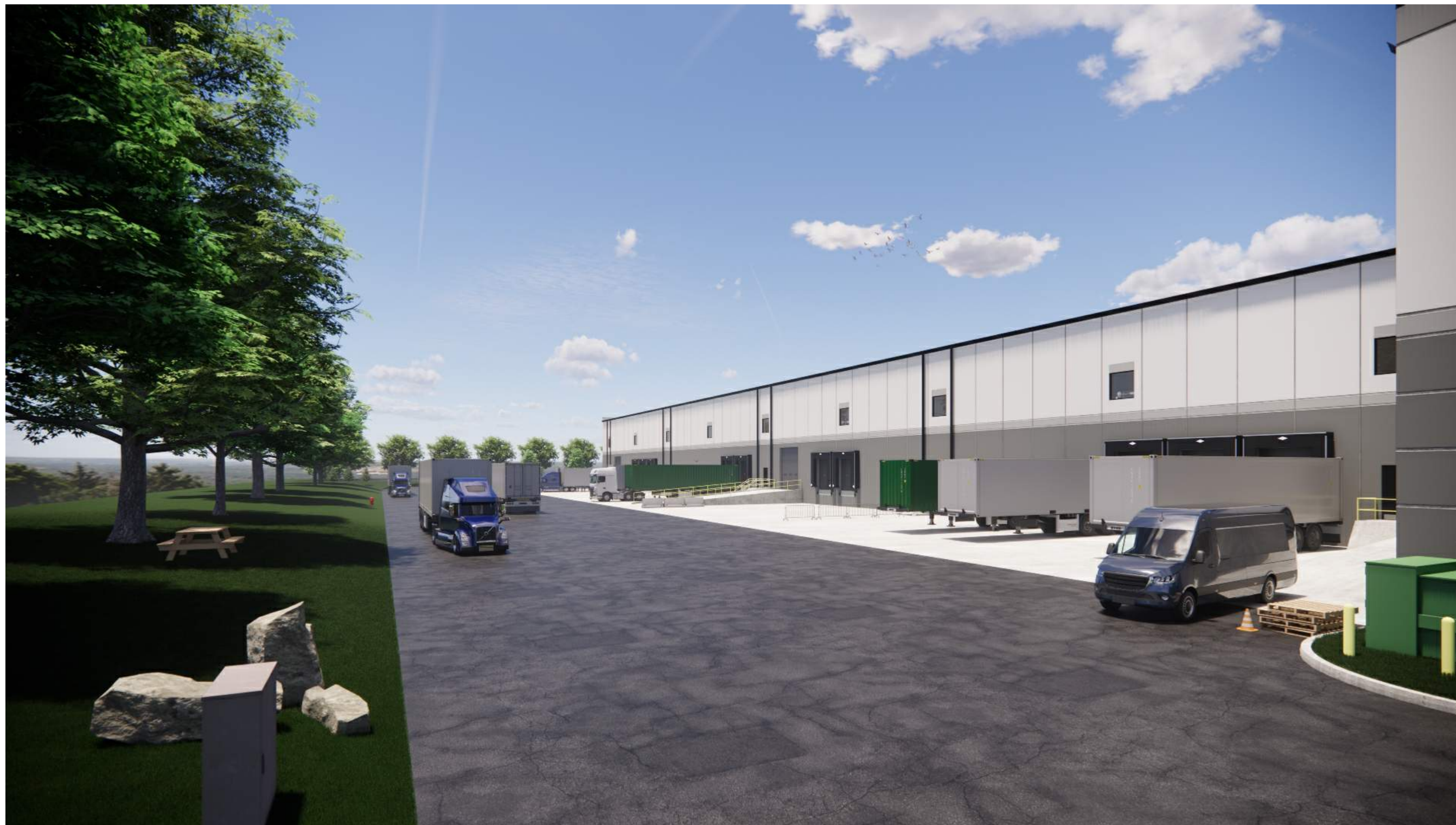
SW Corner - View of Truck Court
