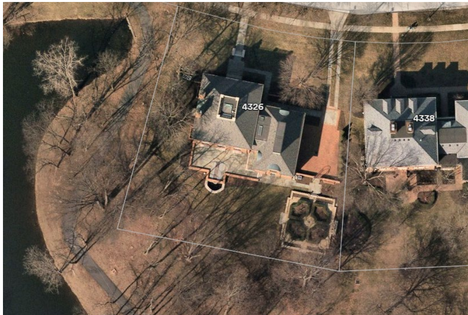
Image: Existing site conditions (March 2024).
