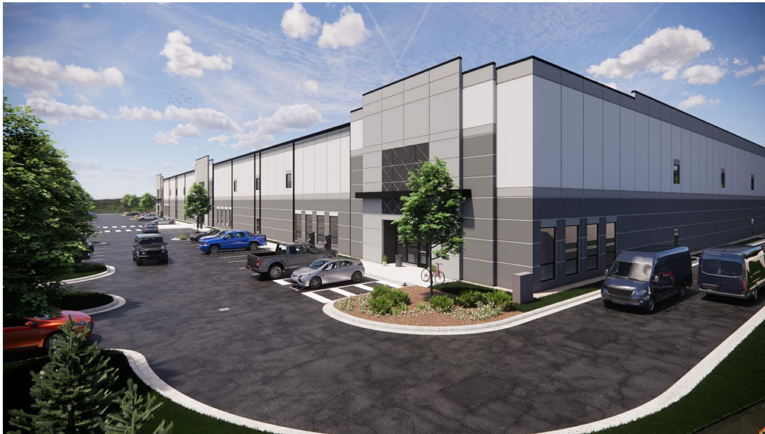
NE Corner - View of Building Entry
