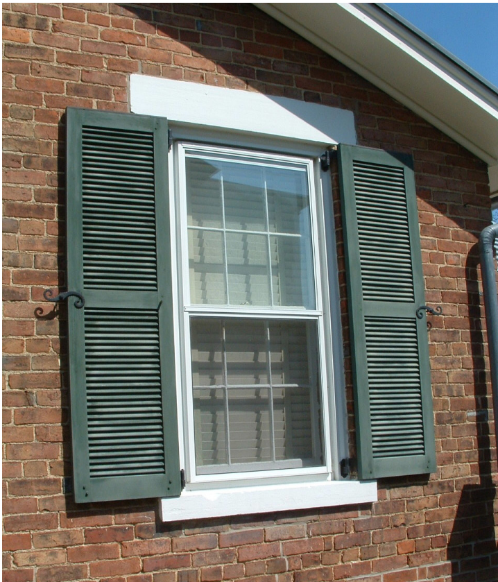
These historic shutters are operable and made to fit the window opening.
