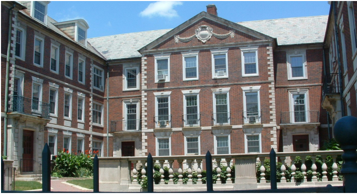
When a courtyard is located within the recessed wings of a building, the entire courtyard may be at least two feet above grade.
