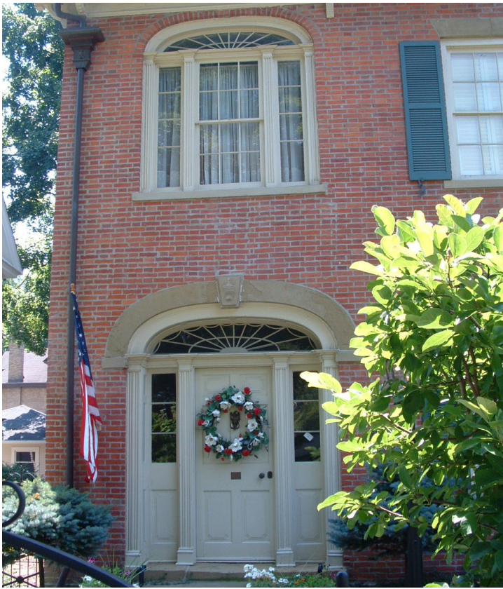
Historic entrances and windows were carefully proportioned and finely detailed.
