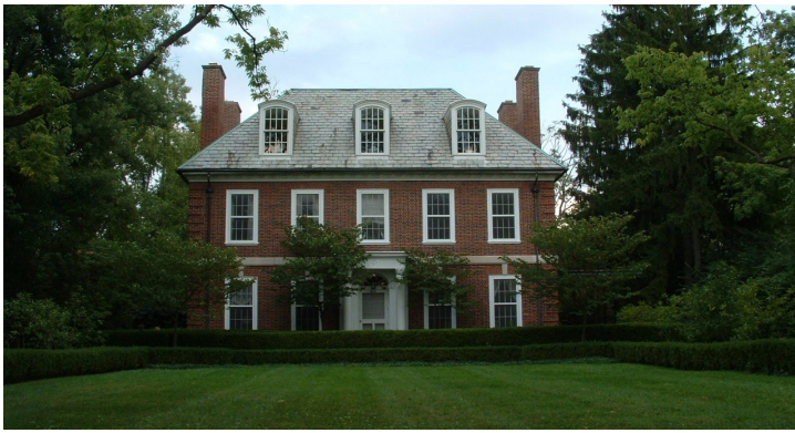
High style designs incorporate specific architectural elements.
