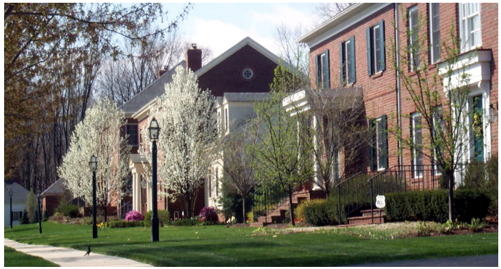
No garage doors face this street, enhancing the feel of a traditional streetscape.
