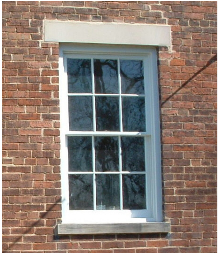
This historic true divided-light window illustrates correct vertical proportions for window panes.
