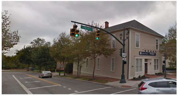
Example of existing Village Center signal mast arm.
