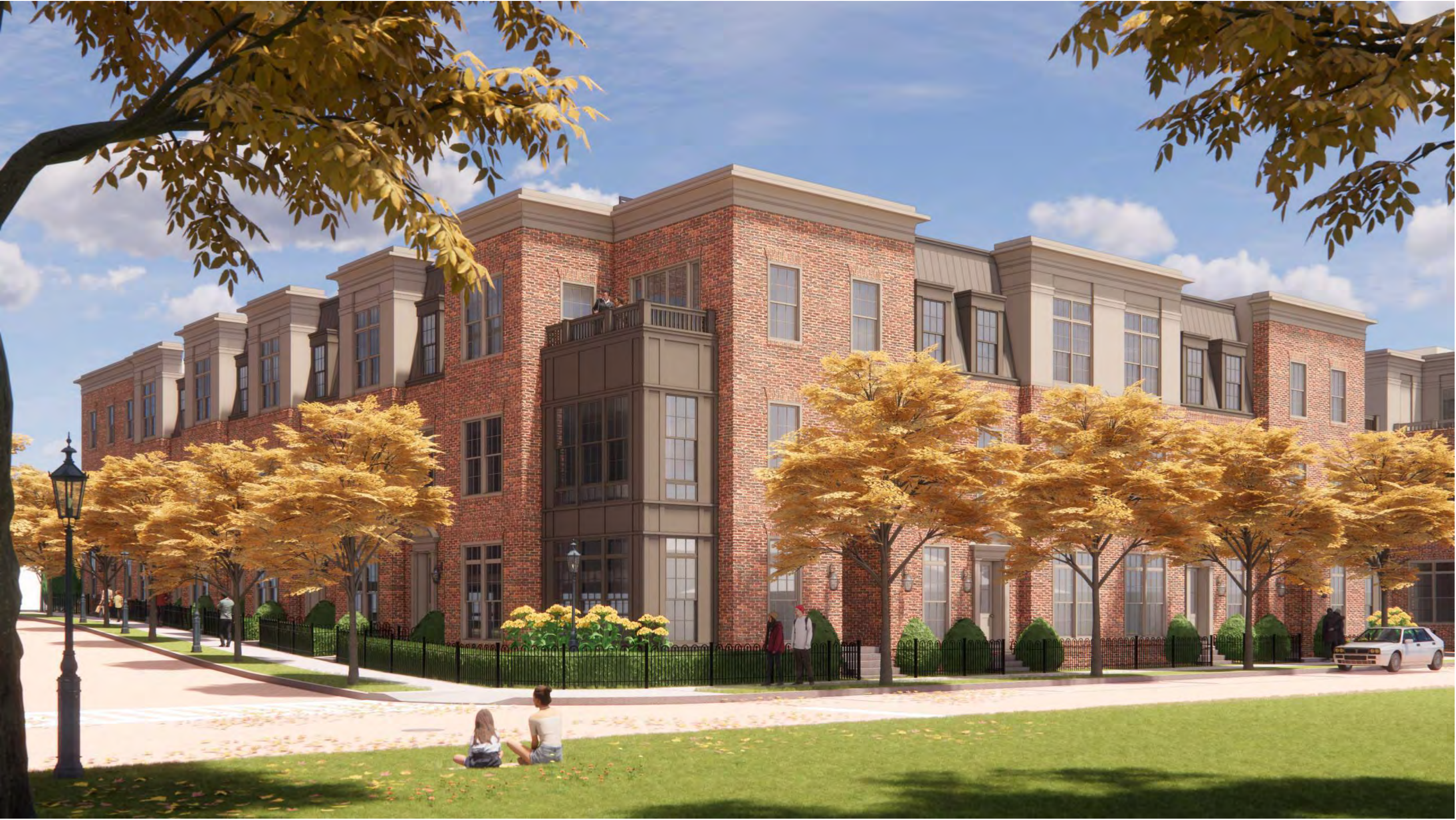
AFTER // Rooftop Garden Access
